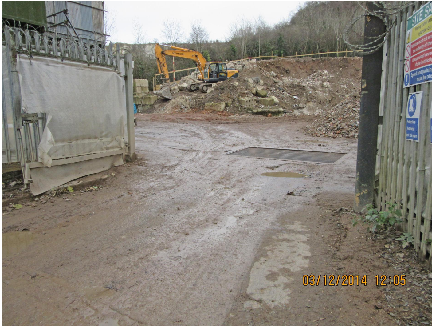
Figure 7 : View looking east, directly into the site from Godstone Road
